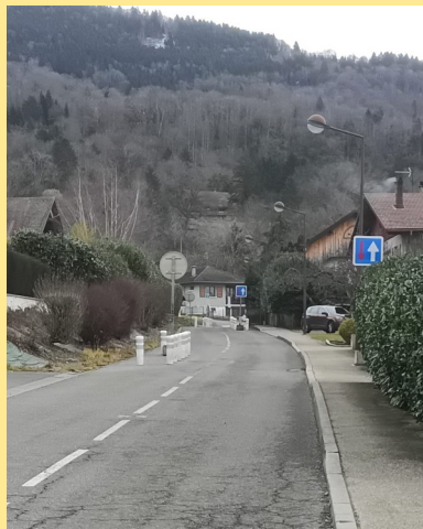
Chicane provisoire, route de la Charniaz
